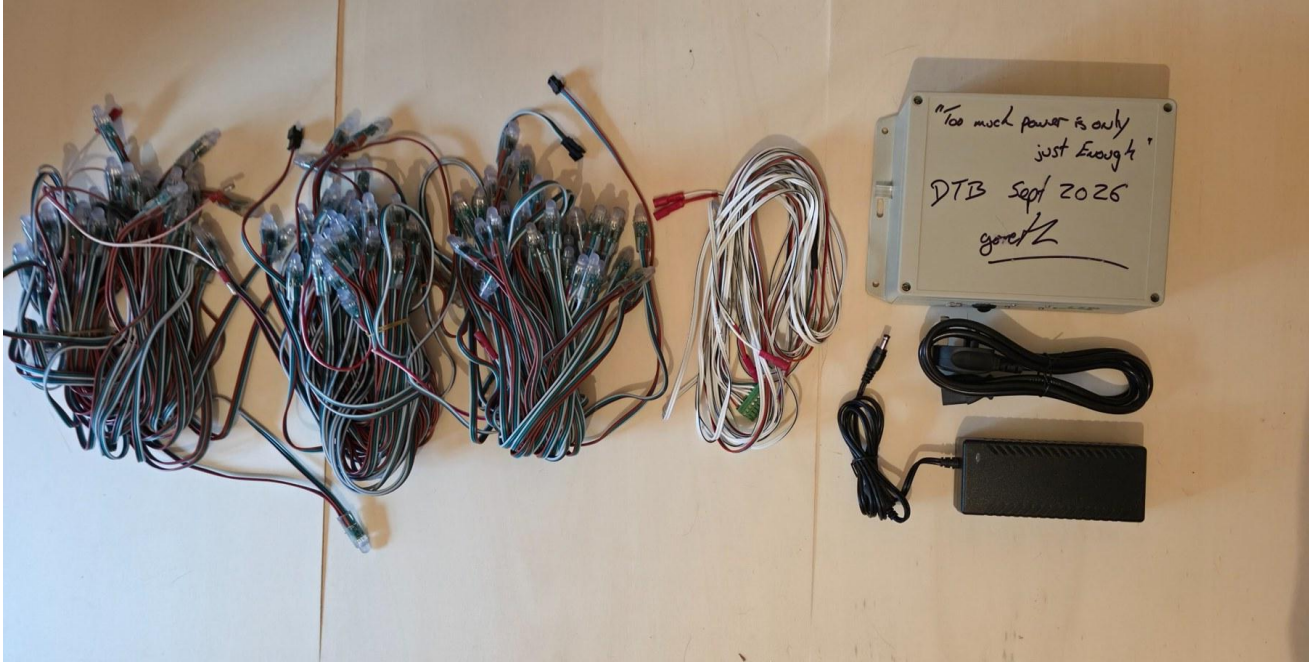
A complete DTB self-install system laid out before fitting the LEDs.
